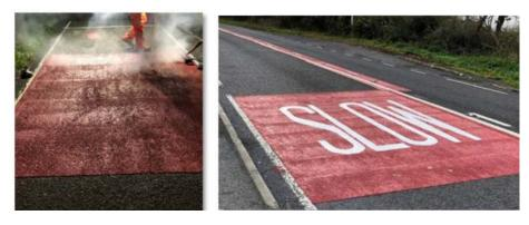
Surfacing and studs after resurfacing the road; the central hatching was also red backed in some areas as can be seen in the picture.
